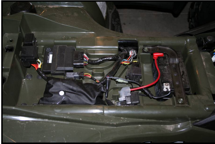
Suzuki King Quad electrical center, Gary Gustafson photo
